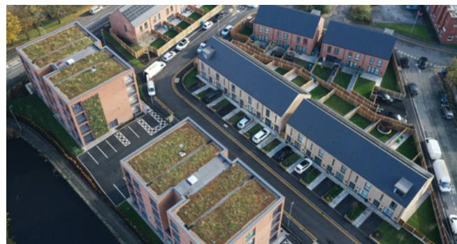
Sixty-nine low carbon homes for social rent have now been completed and residents have been welcomed to their new homes on Silk Street in north Manchester. Image credit: Manchester City Council
